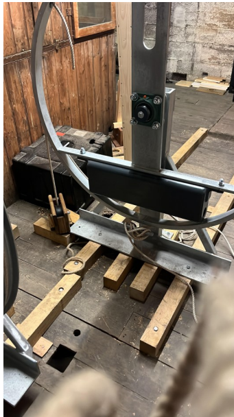
Picture of Training Bells - during installation in the clock room (between the ringing room and belfry)
